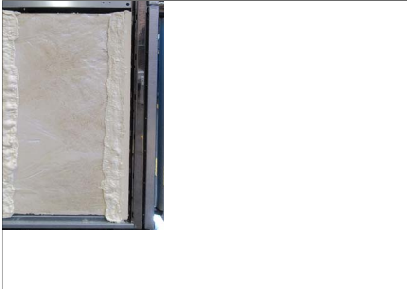
Fig. 1 Pass-through oven UF750TS with wall jamb – view from the cleanroom side
