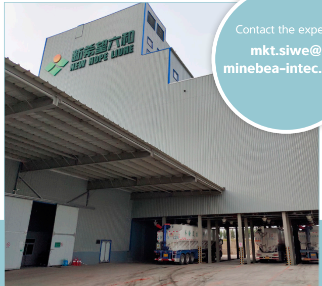
At the New Hope Group site in Liaoning, Minebea Intec successfully installed a total of thirteen truck scales
