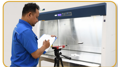
Smoke Pattern Test
