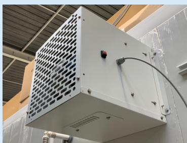
HEPA Filtration with positive/negative pressure
