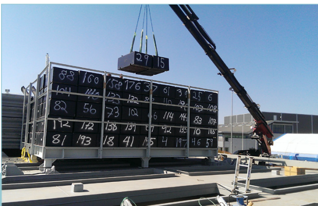
The silo scales were calibrated on the ship with weights of up to 300 tonnes
